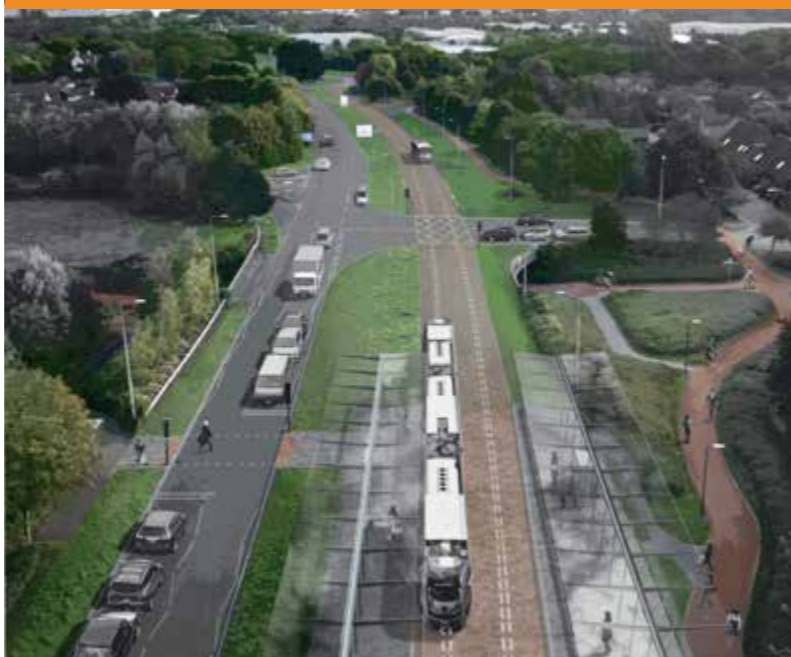
Figure Five An illustration of how one side of a dual carriageway could be used for Mass Rapid Transit services.
