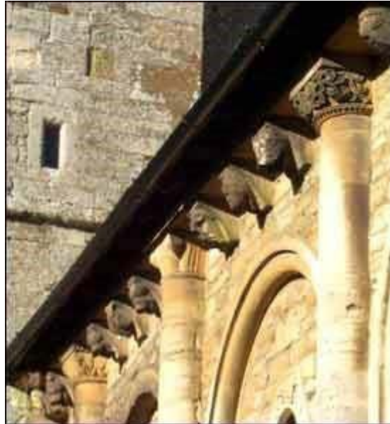
St James church, sunlight shows off the colour of the stone
