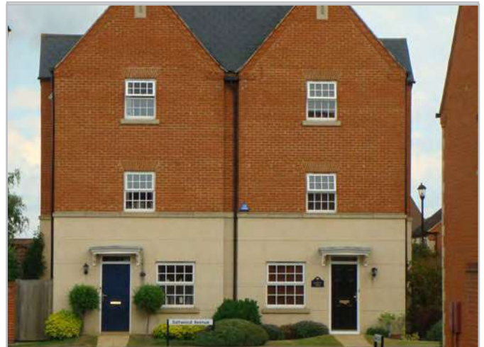
Poor proportion of glazing relative to wall
