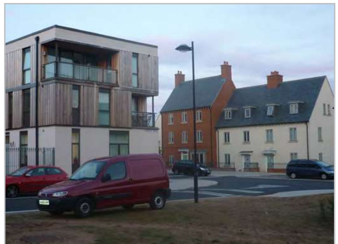
Buildings either side of a street facing each other should not visually clash. The ground floor render in the contemporary building does however at least give some coherence to buildings on both side of the street
