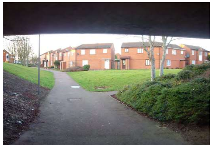
Good surveillance of underpass from neighbouring housing
