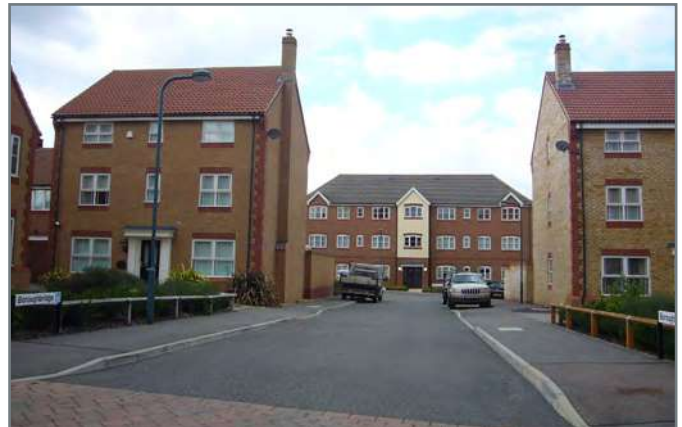
Grange Farm - detailed elevation design has not added to the character of the development
