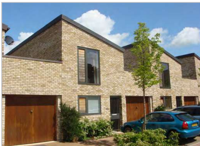
Traditional materials can be used effectively in contemporary designs
