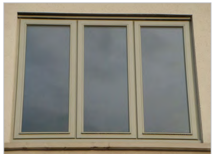
Window frames of different colours should be considered, as they can help create character for a building
