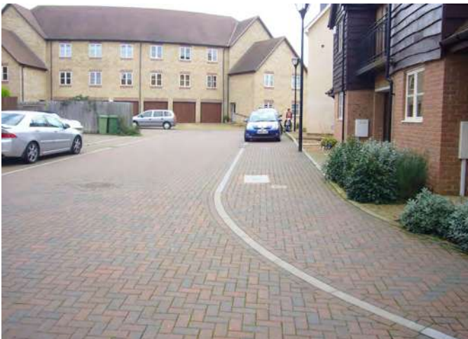
Drainage channels leading to confusion as to whether parts of the level surface are for parked cars or footpaths
