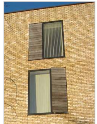
Vertical staggering of windows adds interest to elevation. Alternate material adjacent to window adds further interest
