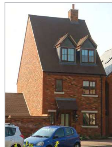
The roof over dominates this house. The location of the dormers furthermore make for poor proportions
