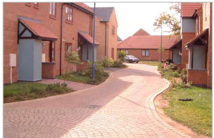
Level surface street too narrow, with poorly defined and overly sinuous edges resulting in vehicles overrunning the carriageway and being unable to pass through when cars are parked in the street.
