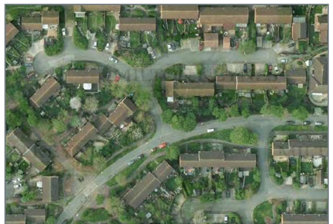
Florin Close, Leopard Drive, Noble Close in Pennyland - buildings positioned to capture solar gain
