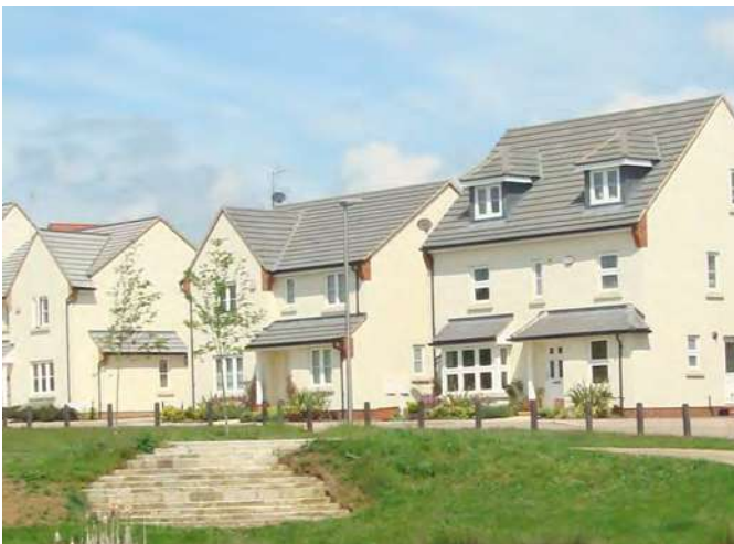
The use of render can create a strong identity for a street: Oxley Park
