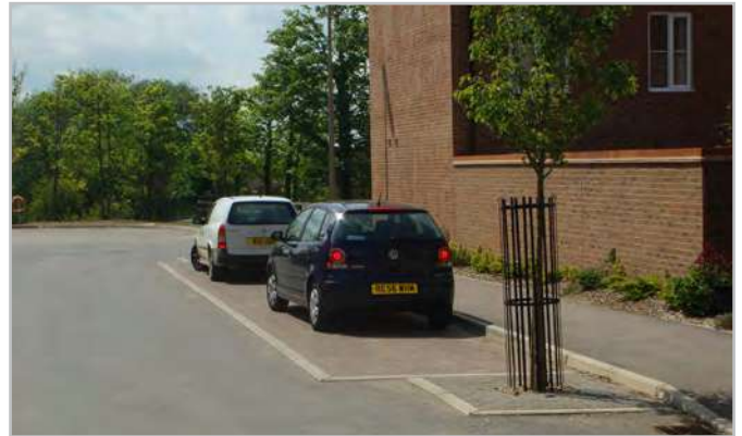
Parallel parking within the carriageway -Woburn Sands
