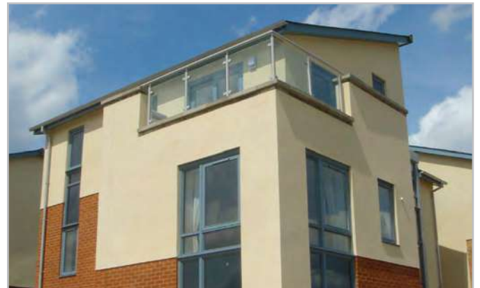
Balconies should be of a usable size and preferably integrated into the building design
