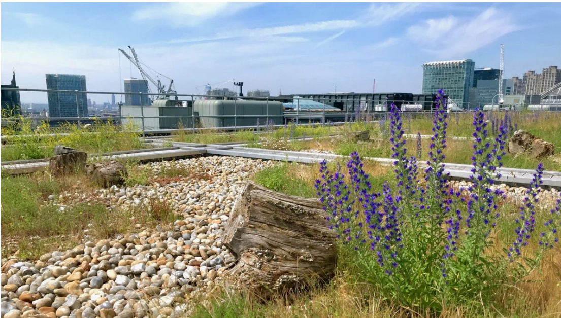
Figure 74: Biodiverse green roof with dry meadow at 201 Bishopsgate, London © Living Roofs
