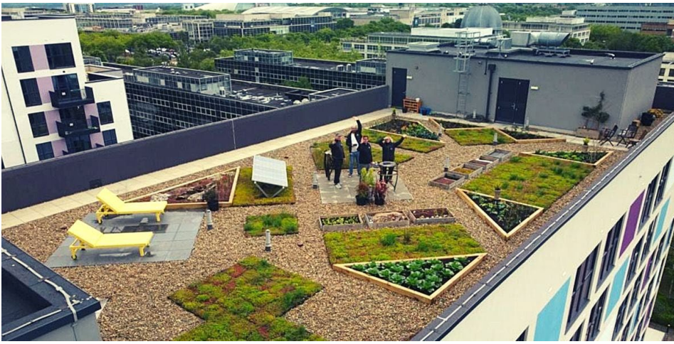
Figure 68: Thin substrate green roof (with raised beds) at YMCA, Milton Keynes © The Green Project
