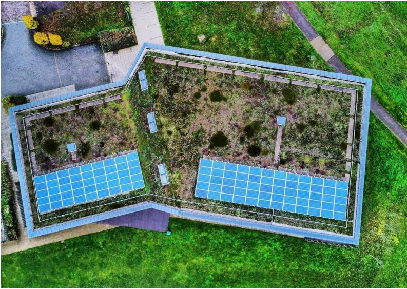
Figure 70: Medium depth green roof at Broughton Pavilion, Milton Keynes © The Green Project
