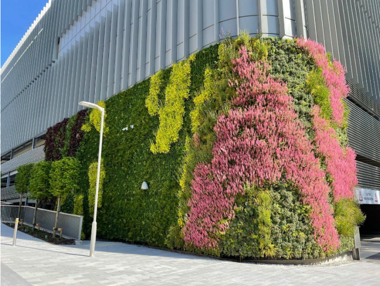
Figure 80: Modular living wall system at Glasshouse Car Park, Cheshire © ANS Global
