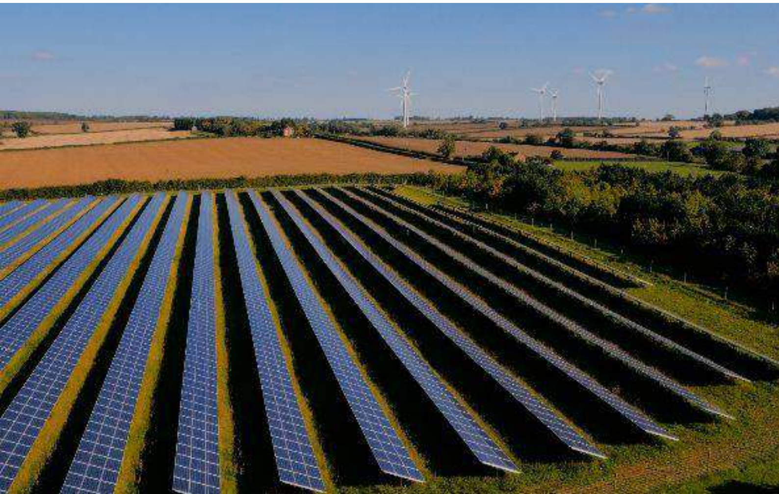
Figure 16: Emberton Solar Farm and Wind Farm
