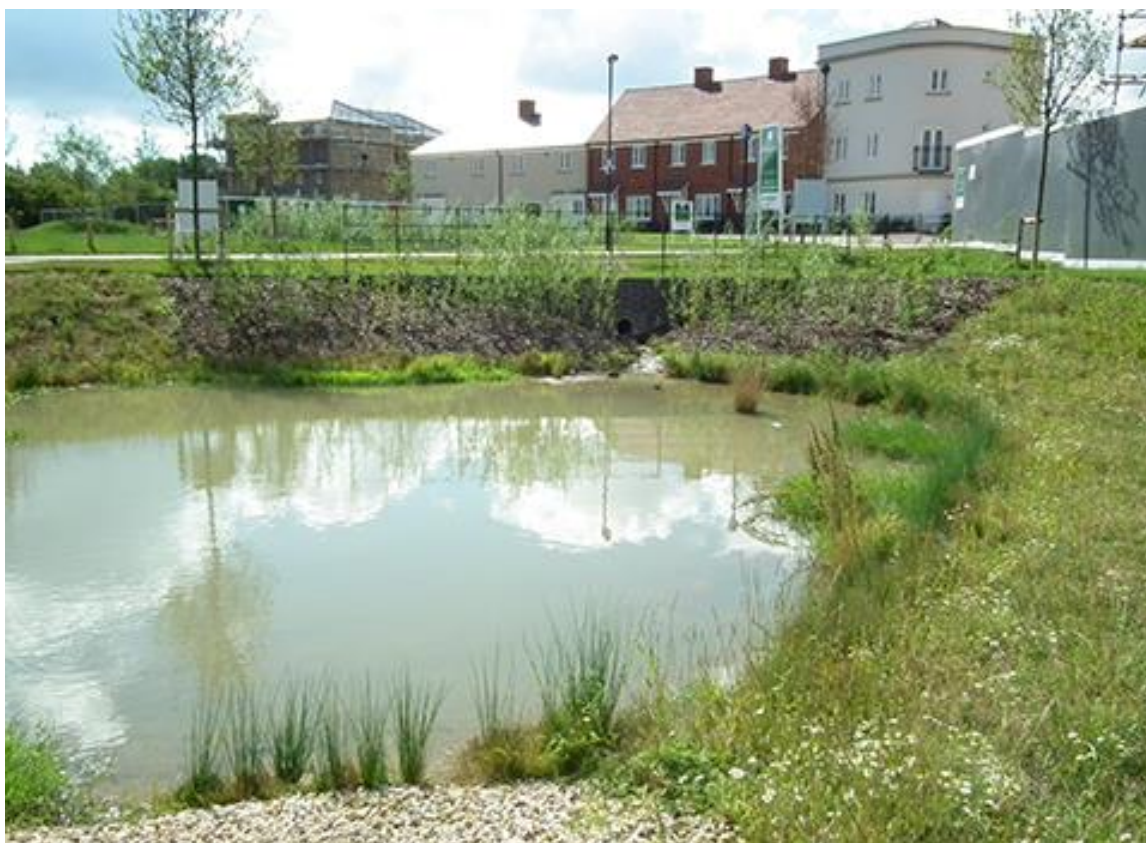
Figure 14: Example of a flood attenuation pond.
