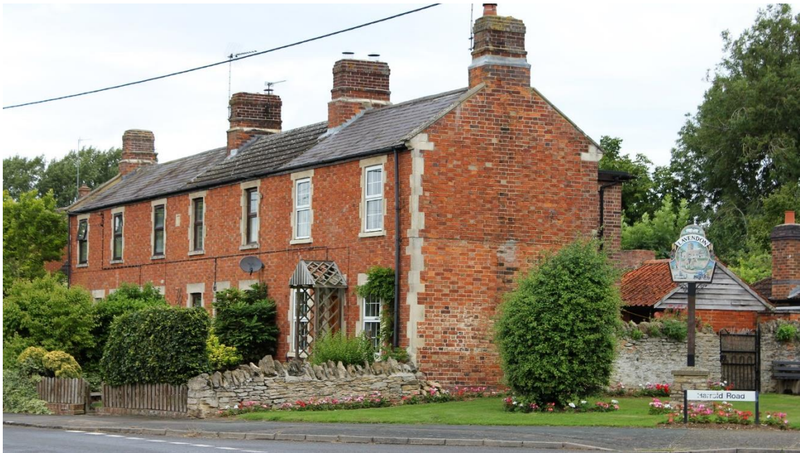
Figure 11: Cottages feature a blend of materials and some fine detailing
