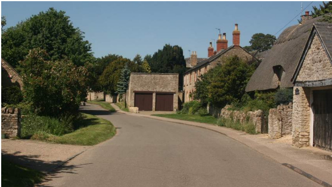
Figure 20: View of Common Street
