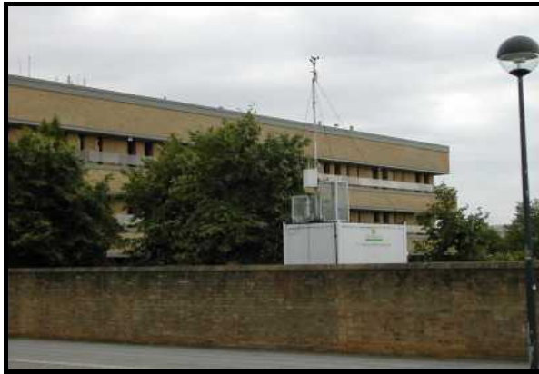
Static Monitoring Station – Civic Offices, CMK (View from North Eighth Street towards Silbury Boulevard)
