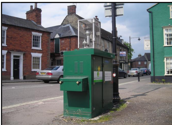
Roadbox 2 Monitoring Station High Street South, Olney (Within Air Quality Management Area)
