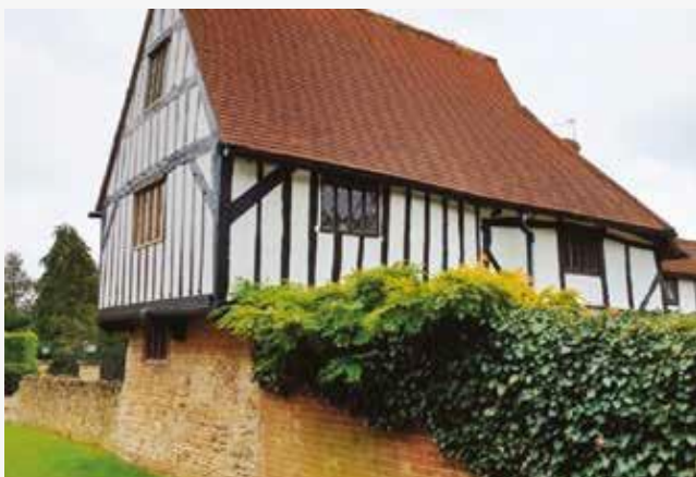
Figure 16: Cillless, side hung, flush fitting, timber windows
