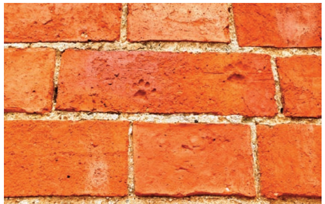
Orange brick with pawprints embedded, set in an offwhite lime and sand mortar with a little hearth grit to aid curing
