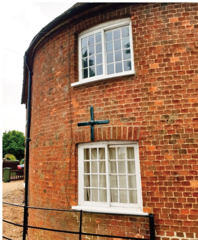
Brick 'headers' used skilfully create a curved wall. The windows are horizontal (Yorkshire) sliding sash that predate vertical sliding sashes. They are of small 12x12 pane puttied into structural (rather than applied) glazing bars under simple segmental brick arches. Some old glass survives and the impressions for a hinge that supported a shutter are still observable.
