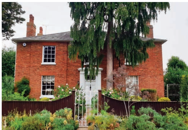
Timber doors and windows set in a symmetrical brickwork composition under a Welsh slate roof. The windows are 'six over six' timber vertically sliding sashes whilst the front door is of eight panels under a fanlight (or 'transom' light) and set within a restrained early Victorian door surround. Note the relatively small size of the door in the context of the ornamental treatment and the ornamental iron gate.
