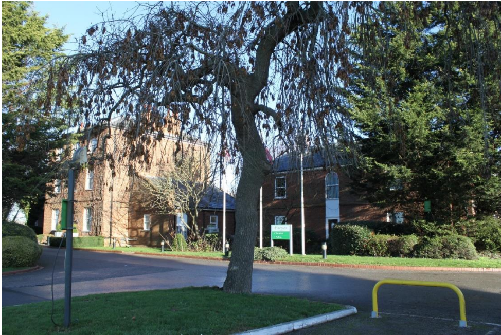
Figure 6.60: Holiday Inn hotel – former Moulsoe Buildings Farmhouse
