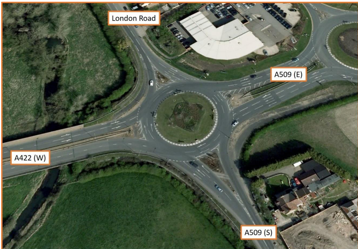
Figure 13: existing Tickford Roundabout
