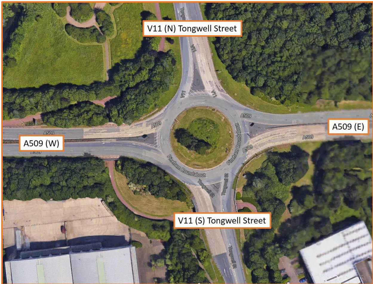
Figure 16: existing Pineham Roundabout
