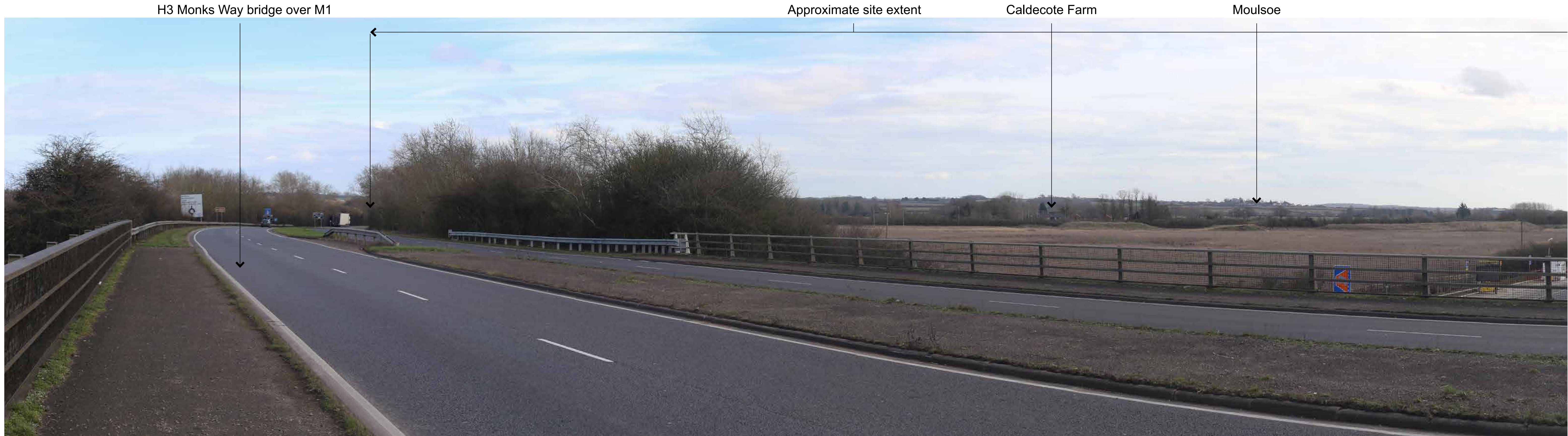
Photo Viewpoint 8: View southeast from A422 (H3 Monks Way) bridge over M1
