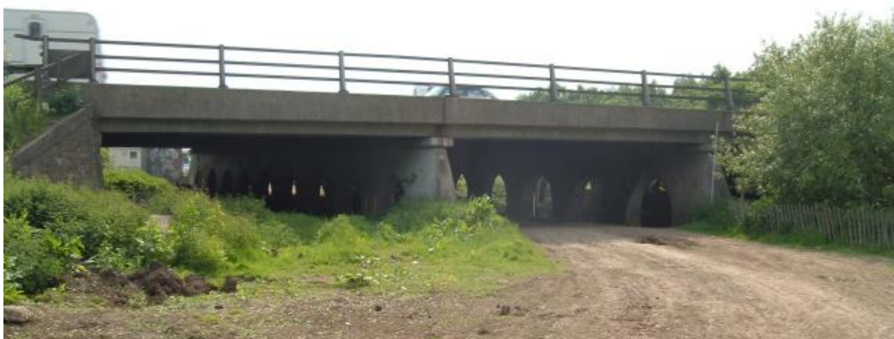
Figure 9 - River Ouzel beneath the M1, showing tie into highway embankment (downstream – right bank)
