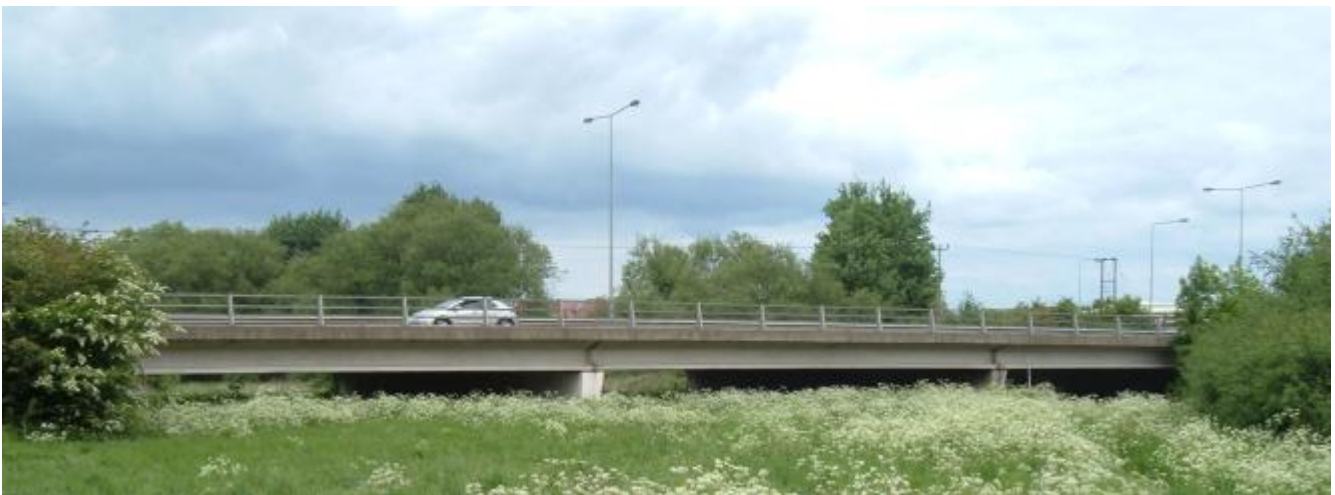
Figure 11 - A422 Floodplain Opening (close view)
