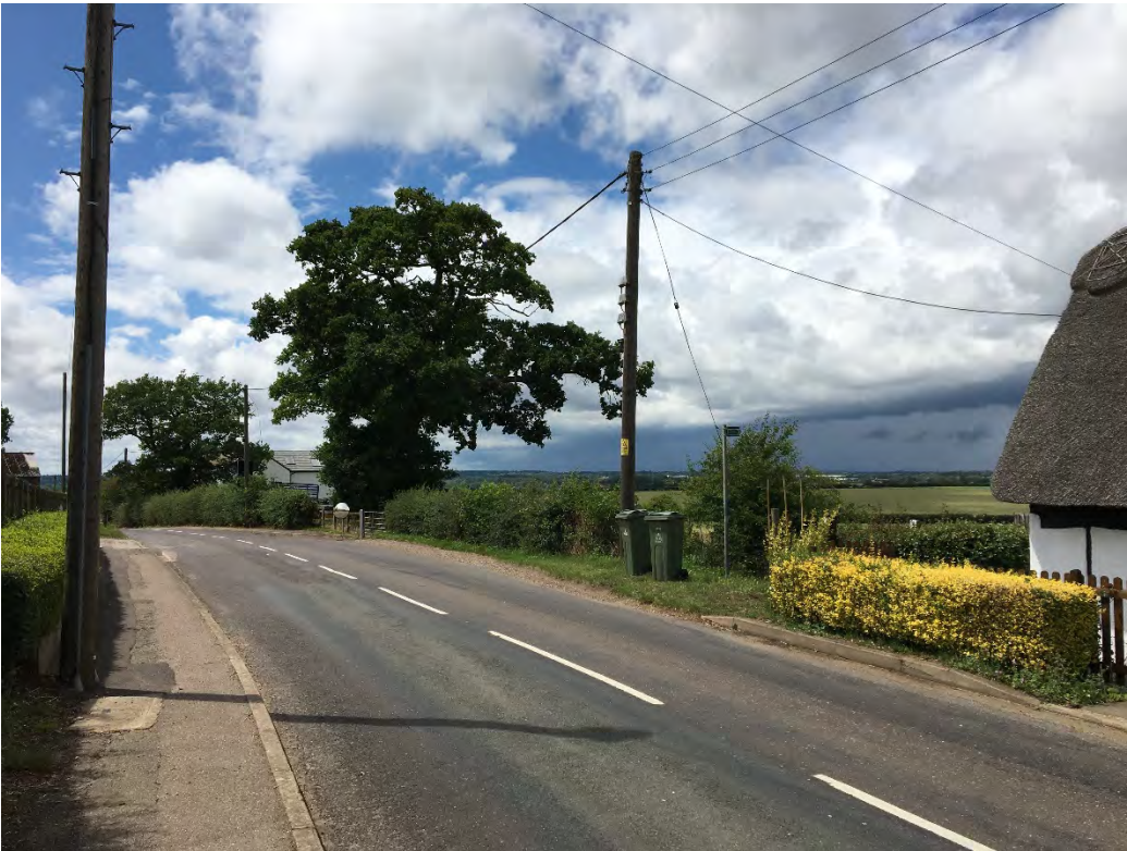
Figure 21: The elevated position of Moulsoe in the landscape is such that it benefits from wide ranging views westwards towards the Site. Listed buildings along the western edge of Newport Road would experience distant visual effects of development within the Site, which would be mitigated through an appropriate landscaping strategy.
