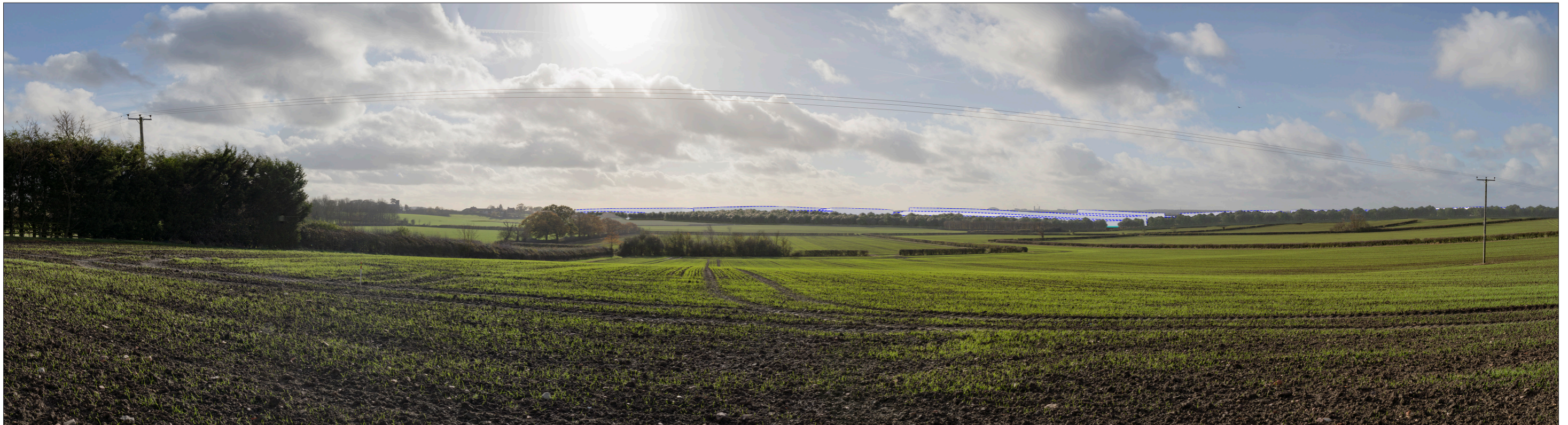
PANORAMA TAKEN FROM VIEWPOINT M10 REPRESENTING PLANTING 15 YEARS POST COMPLETION (2062) - ALLOWING FOR A FURTHER 15 YEARS OF TREE GROWTH AT A RATE OF 300MM PER ANNUM AND A MATURE HEIGHT OF 15M. THE FOLLOWING ELEMENTS OF THE SCHEME ARE VISIBLE: DEVELOPMENT ENVELOPE (BLUE DASH OUTLINE) AND THE EDGE ROAD WHERE IT CROSSES THE MOULSOE STREAM(CYAN OUTLINE)
