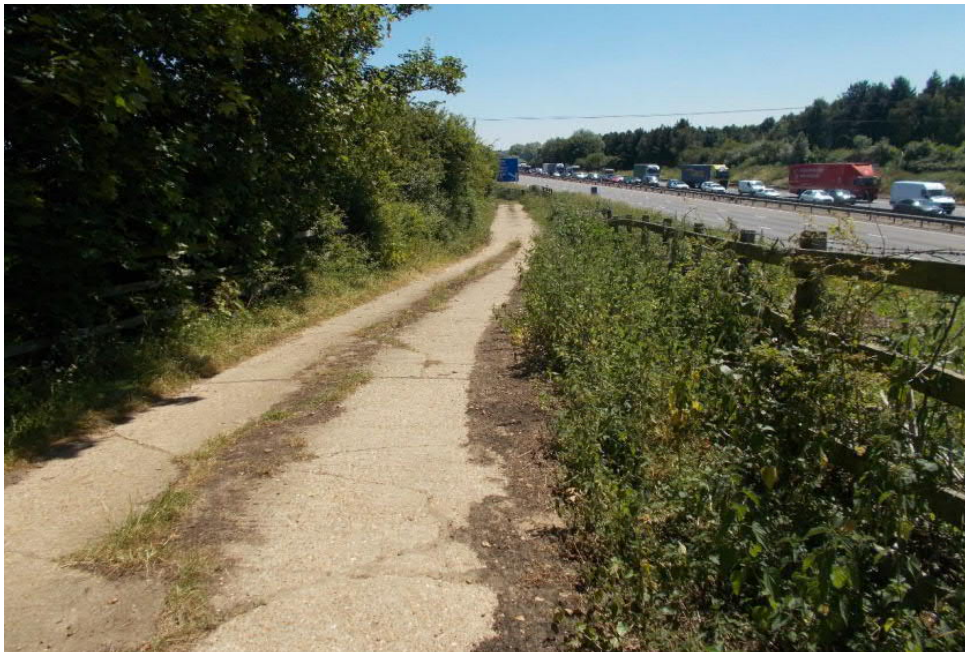
Photo 5.2 – Accommodation bridge northern ramp – looking southeast
