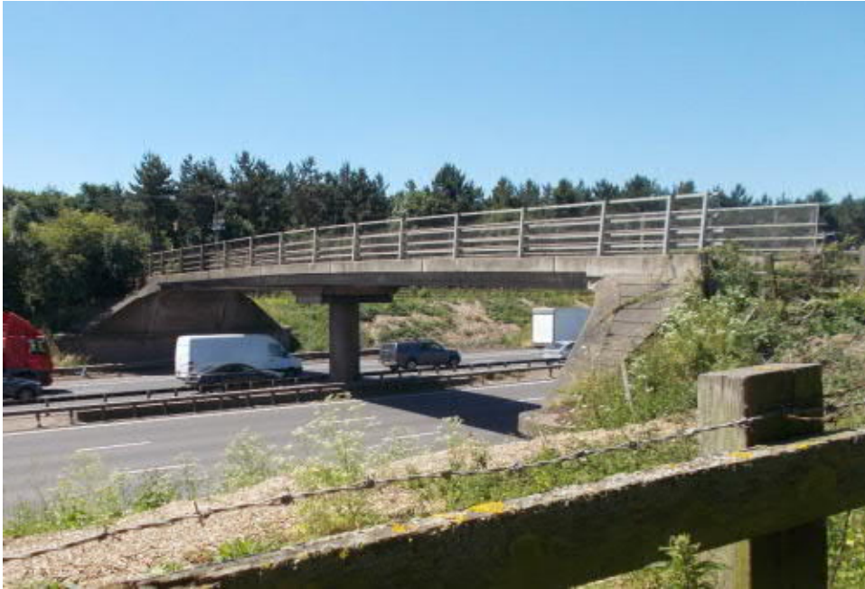
Photo 5.1 – Accommodation bridge – southeast elevation
