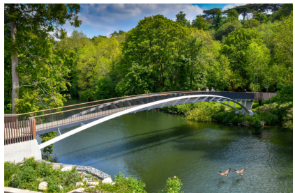
Pedestrian Bridge at Horsham - Berkeley Group
