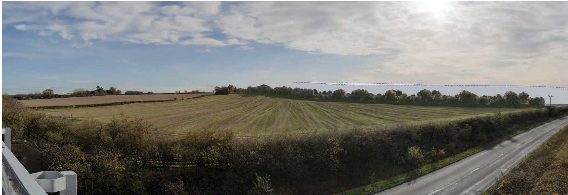
Panorama taken from viewpoint L8 representing planting at completion of the scheme (2048) - allowing for 18 years of tree growth at a rate of 300mm per annum
