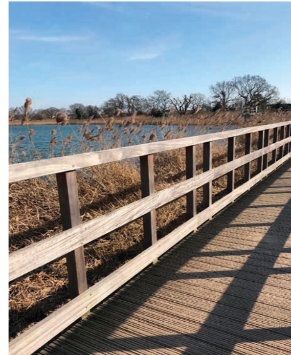
Timber boardwalks and bridges
