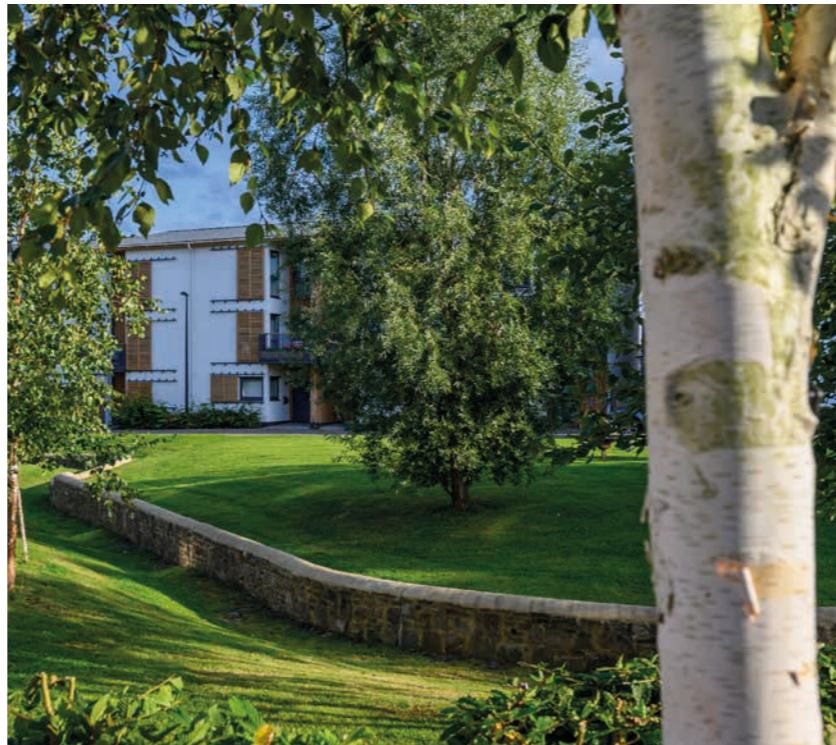
Swale with natural stone wall, Hanham Hall
