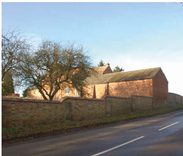
Agricultural building on Newport Road, Moulsoe
