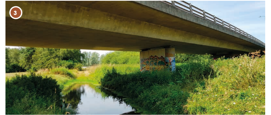
3 River Ouzel flowing under the elevated M1
