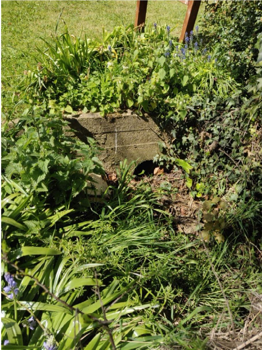
Figure 3: Harrold Road Culvert
