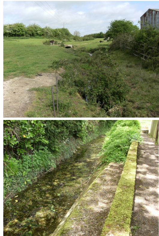
Figure 7-3 Examples of Milton Keynes Watercourses Requiring Enhanced Maintenance.
